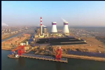
2X660 MW PORT QASIM
