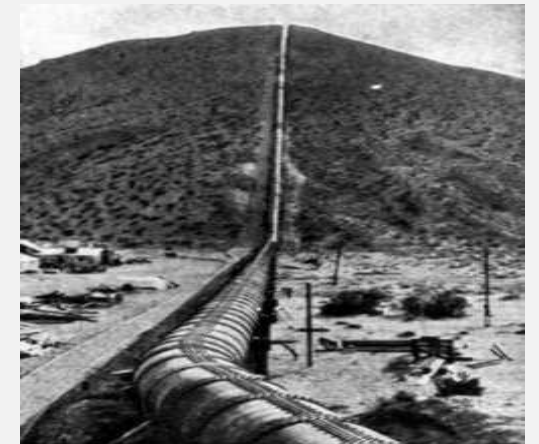
Pipeline in early ages
